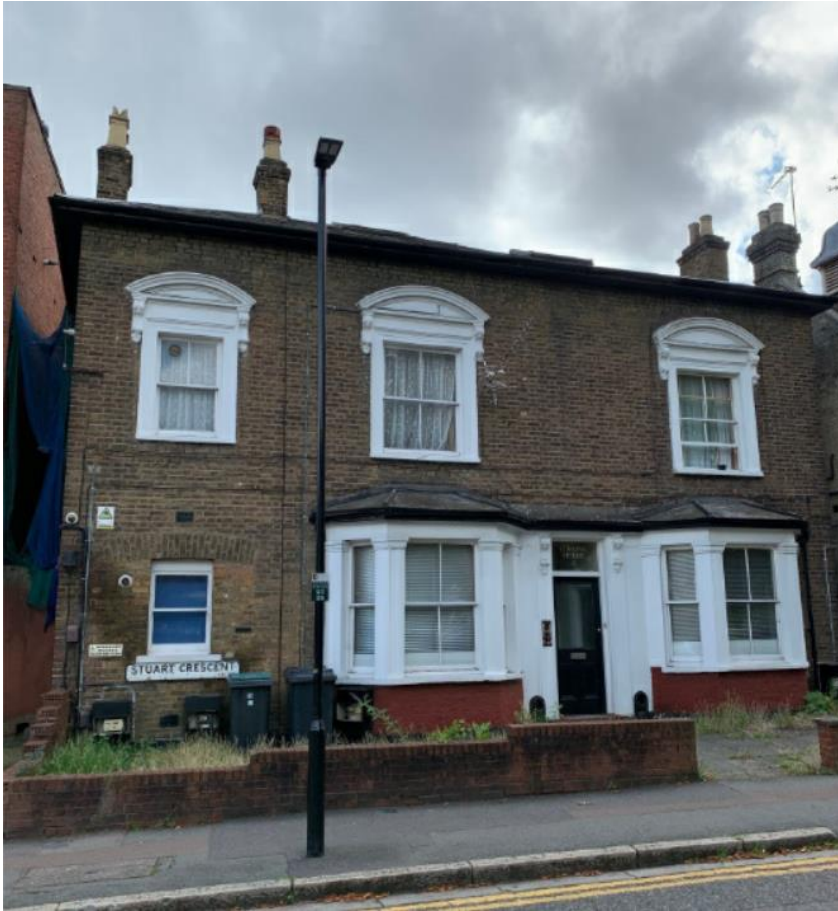
Figure 3: – Existing Social Club (Locally Listed) Building – flats at first floor
